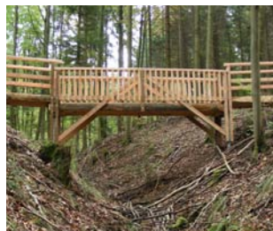
Timber bridge, Baden-Württemberg
