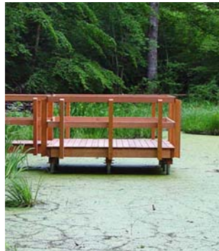
Bird-watching footbridge (Switzerland)
