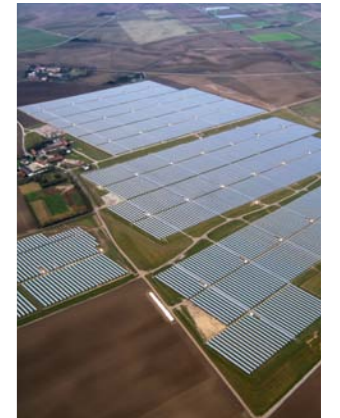
One of the globally largest solar farms (54 MWp), Gänsdorf
